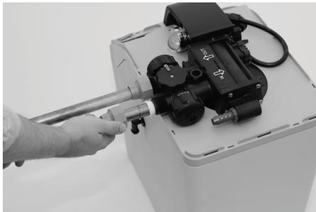
**Diagram 9:** Connect Water Lines (Shown with Bypass Valve)
